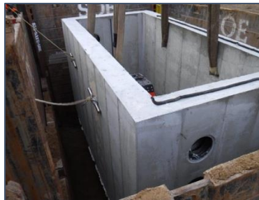
Vault Installation
